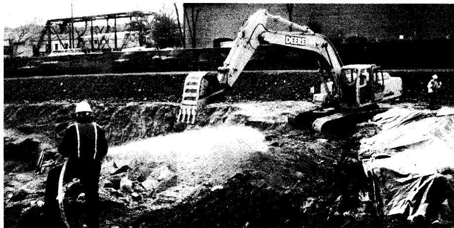
A worker sprays water to control dust as heavy equipment excavates soil at the site.
